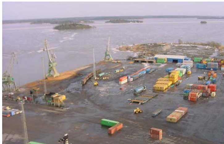
Picture on new harbour quay in Västerås, Sweden
