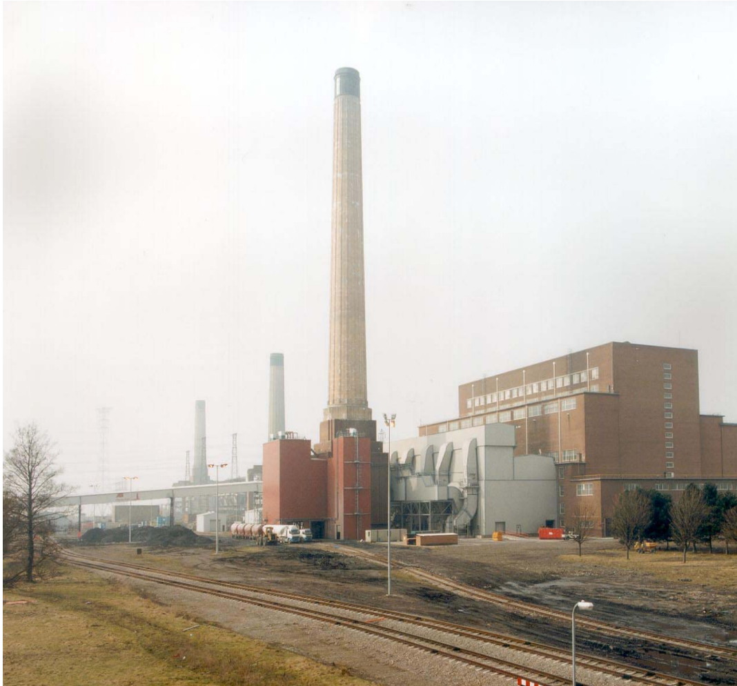
Uskmouth Power, Unit 13, 14 & 15, 3 x 120 MWe
